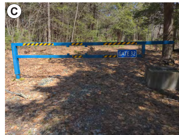
The entrance to the Springfield Water and Sewer right-of-way
