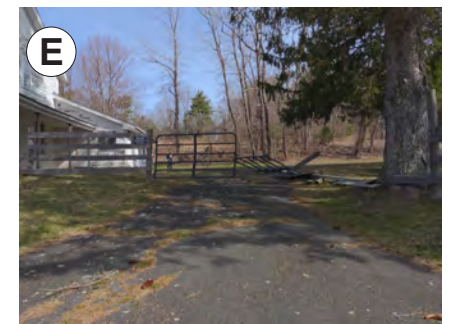
The steep, gated driveway limits safe access to the meadow from Otis Stage Road.
