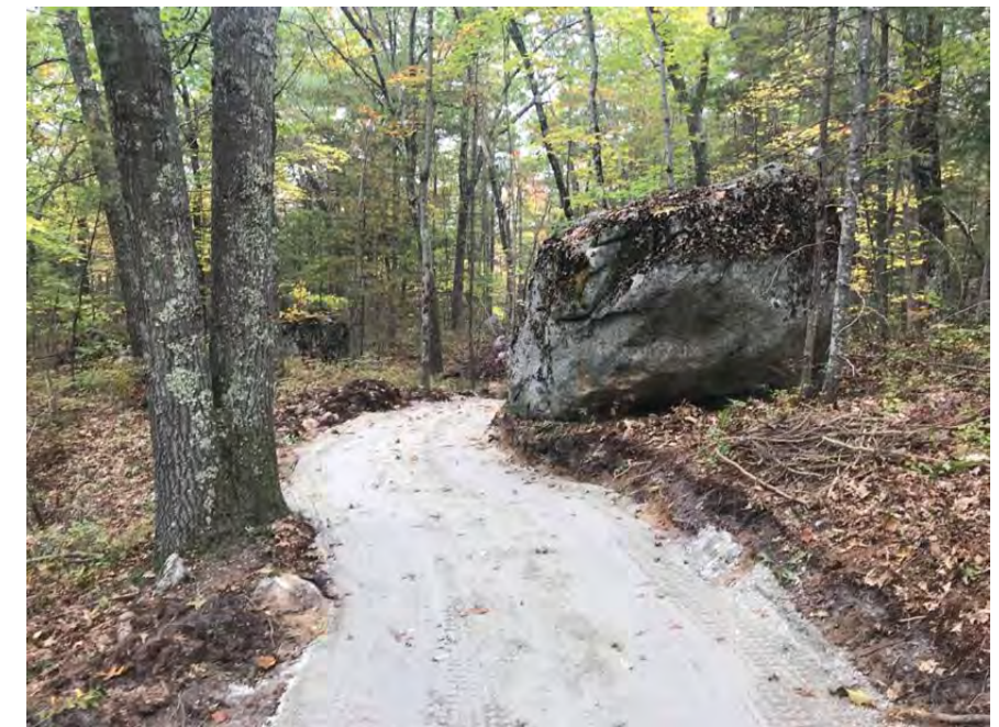
All-Persons Trail in Manchester, NH; design incorporates existing structure, such as boulders and trees, to anchor the trail in the landscape; firm and stable materials allow for universally accessible travel.
