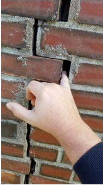
1 Fire Garage exterior wall, 2018. Photo Credit: Ed Harvey, Former Fire Chief, Town of Blandford
