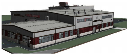
As the OPM Project Director, David Shrestinian has been working closely with the design team on the Town of Rockport's DPW facility.
