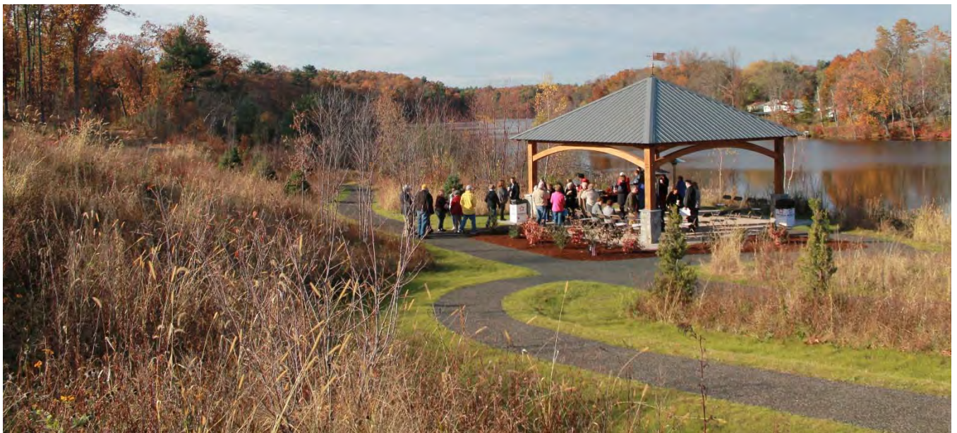
Timber frame pavilion at Gunnery Sgt. Sullivan Park
